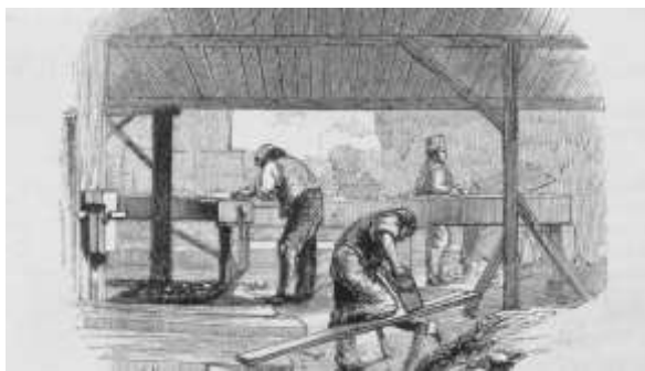
The Carpentry Shop
